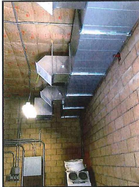
Installed ceiling insulation and AC air ducting
